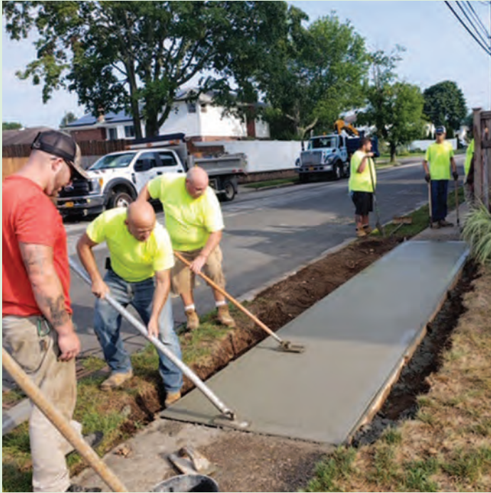
Town of Babylon DPW Mason Crew floating and creating contraction joints in the newly poured sidewalk for residents in Deer Park.
