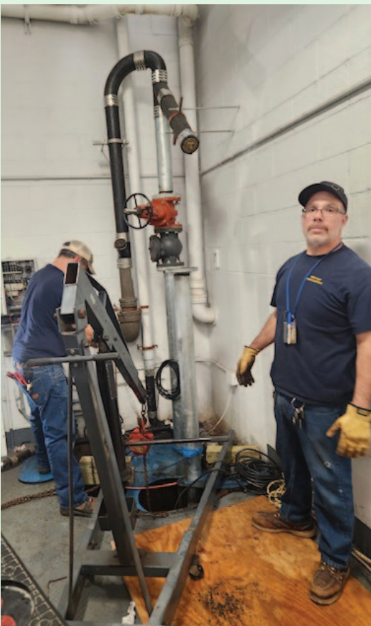
West Islip School members Troy Trabacchi and Bryan Accettella removing a bad trash pump, fixing it and installing it. These guys are very skilled and save the taxpayers money by doing it in house. Great job!
