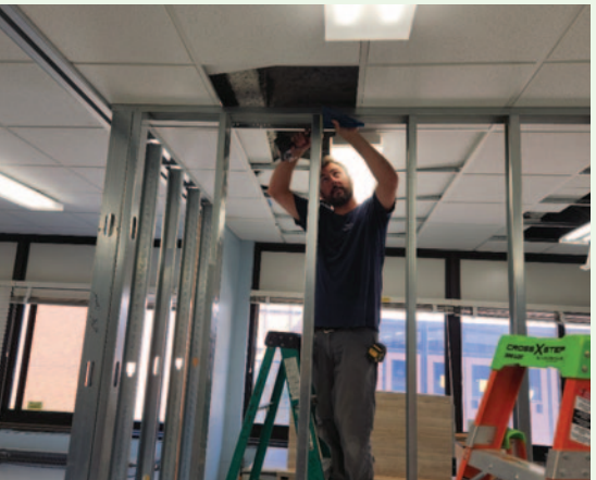
West Islip Maintenance Shop doing major renovations, framing offices for the I.T. Department. Framing, electric, sheetrock, spackle, paint and doors. Skilled members who do most work in house. Great job Teamsters!
