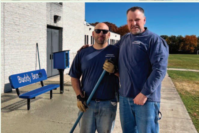
Commack Teamsters pouring and finishing cement at Burr Intermediate School. Head Custodian Todd Raplee , Adam McCabe and Rich Bullis all did a great job! This is a part of a memorial dedication for a former student.
